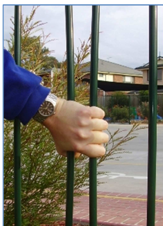
An example of non-conforming playground fencing due to excessive flex in the picket
