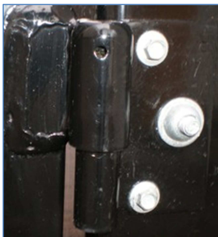
Goliath (ball bearing) hinge
