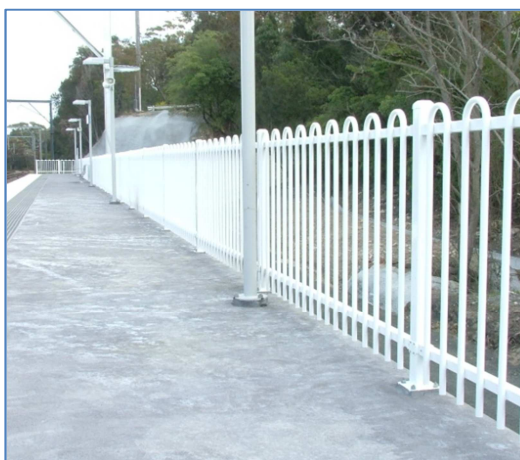
Loop top (railway platform)
