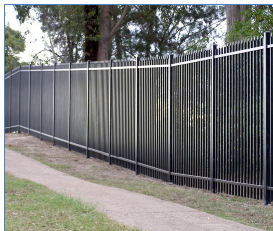
Raked fence panels to maintain clearance under the fence
