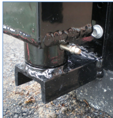
Heavy duty hinge with greasable tapered roller (thrust) bearing
