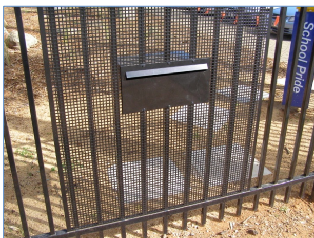
Letter box (anti-climb design) set in a perforated mesh panel
