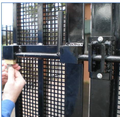
Broadhurst lockbox and Ø20mm slide bolt
