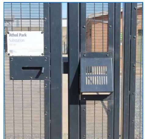
Slide plate anti-climb and vandal resistant hand-hole arrangement for sliding gate
